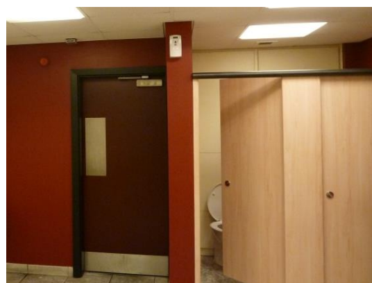
Figure 5: Toilet inside door and exit route
